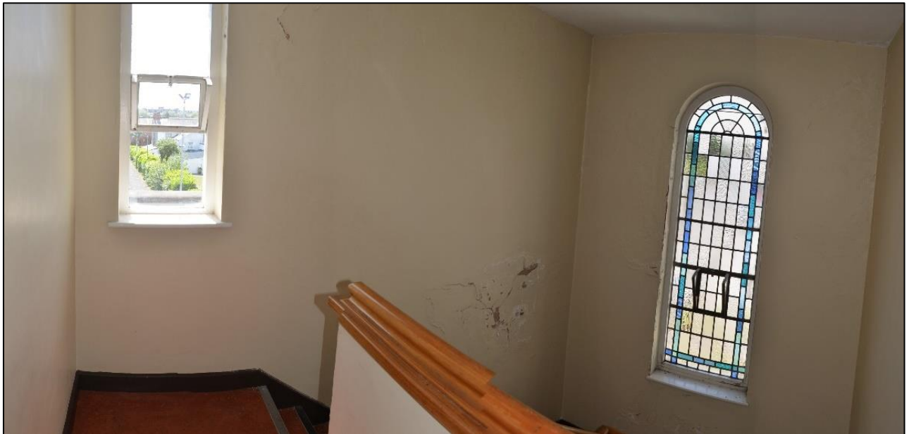
Figure 14.58: Front stair hall to the building.
