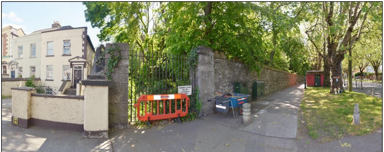
Figure 14.38: View showing Nos. 133 and 135 Drumcondra Road Lower, with the subject gateway to the right.
