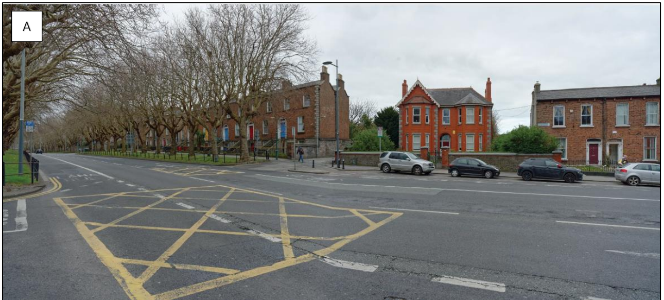
Figure 14.82: Baseline (A) and proposed (B) cumulative viewpoints showing the houses along Drumcondra Road (Protected Structures). View No. 25, prepared by BSM.
