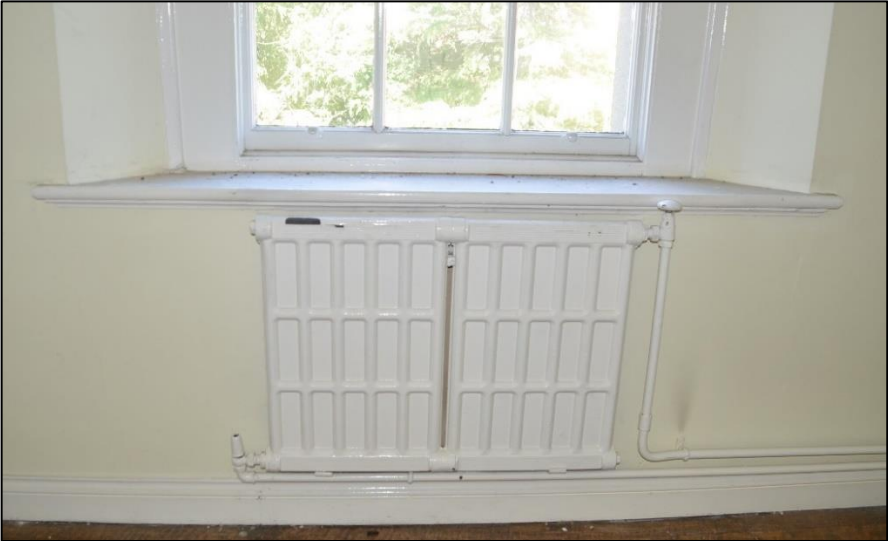
Figure 14.61: Photo showing a surviving cast-iron radiator within the New Wing. There are several surviving examples of this type of radiator throughout first and second floor levels.
