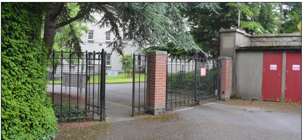
Figure 14.39: Gateway between Archbishop's House and Holy Cross College
