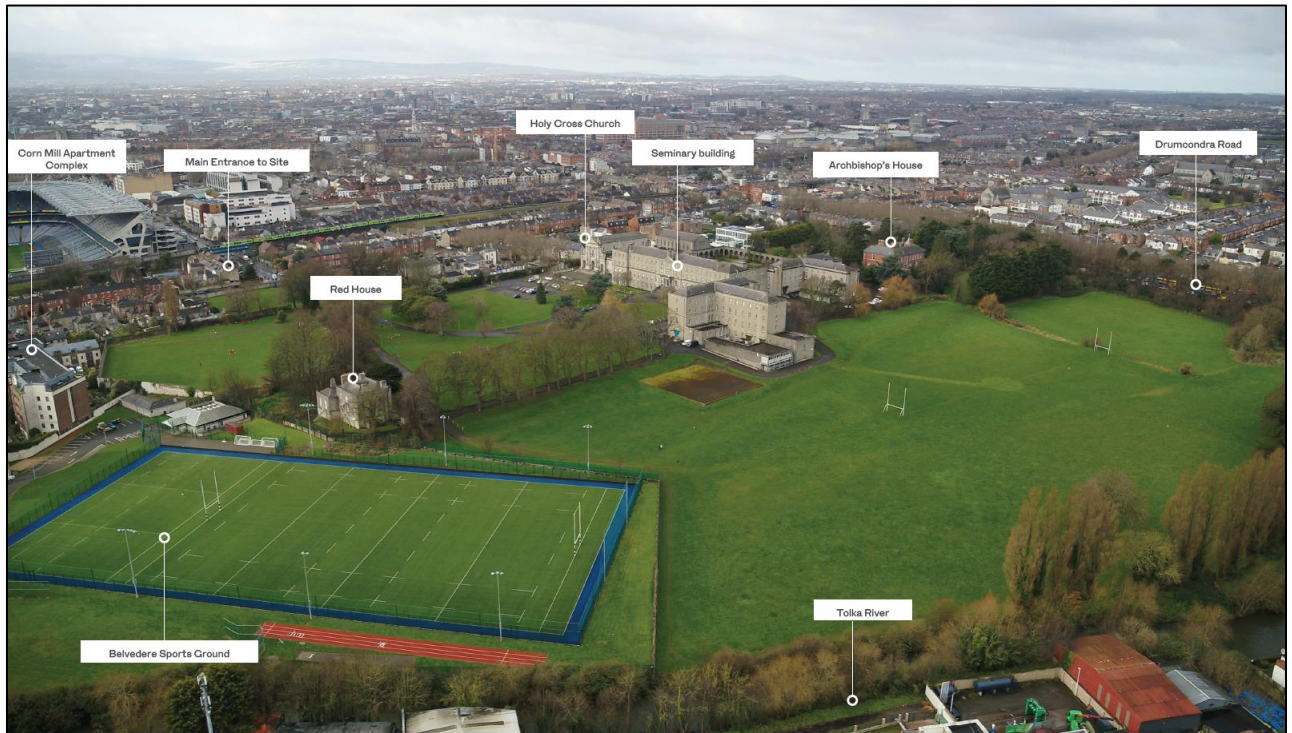
Figure 13.2: Aerial View south-southwest over Holy Cross College lands (Site Strategy Document (HJL 2021))
