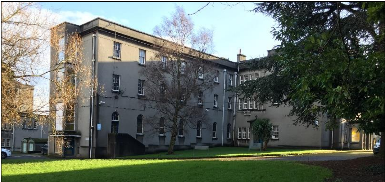
Figure 15.8: Central buildings, facing southeast
