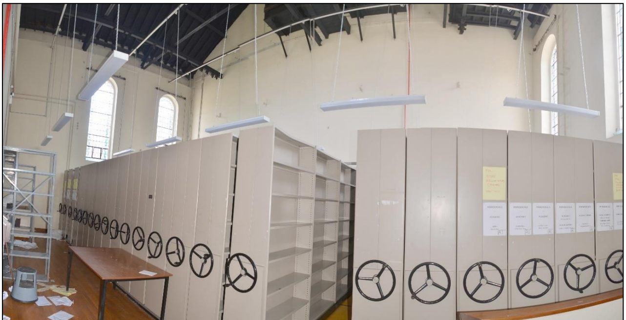
Figure 14.59: Room to the rear of the building, formerly where the stage was located.
