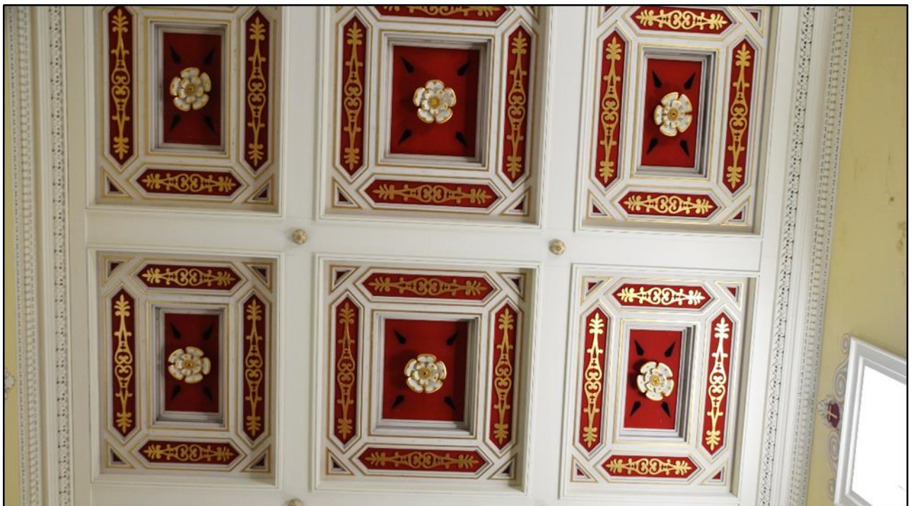
Figure 14.50: View of the panelled timber ceiling to the nave of the Church.
