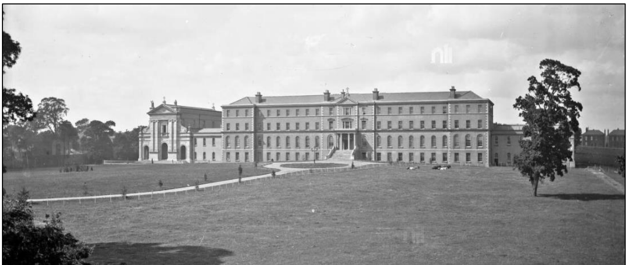
Figure 14.70: Late 19th Century Photo of the front setting of the Main Block and Church. NLI_L_ROY_01108.
