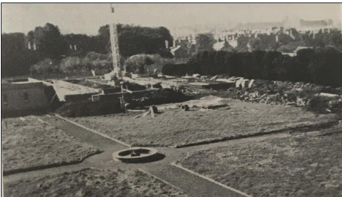
Figure 14.20: Photograph showing the construction of the new Assembly Hall.
