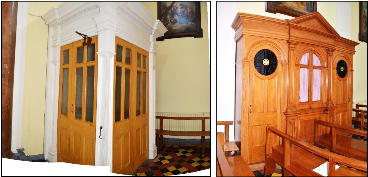
Figure 14.51: Internal timber entrance porch (left) and timber confessional box (right).
